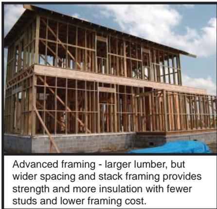
Advanced framing - larger lumber, but wider spacing and stack framing provides strength and more insulation with fewer studs and lower framing cost.
